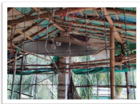
11. THE CEILING OF DEY POULTRY, MADE OF POYTHENE, BAMBOO TO KEEP
